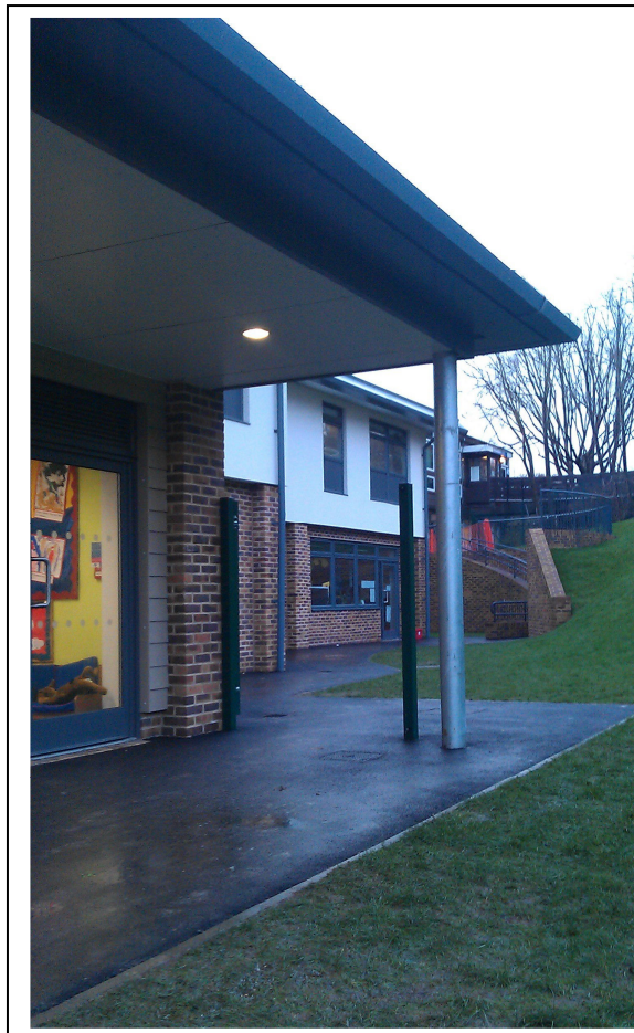
Westdene Extension completed 2012
